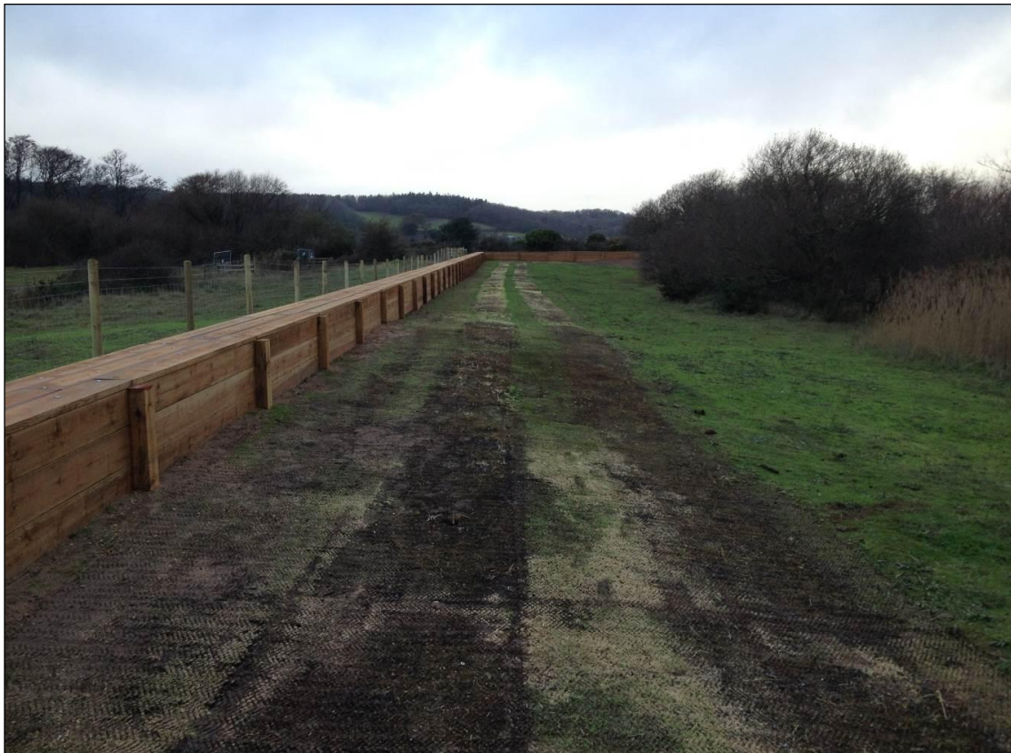
Photo 1. New timber clad flood defence wall
